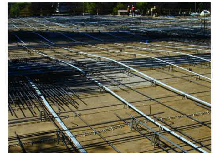
(b) View of a post-tensioned slab (P139)
