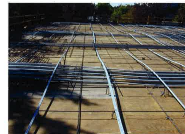
FIGURE 4.8.8A-2 View of a Banded-Distributed Tendon Layout, Using Unbonded Tendons (P328)
