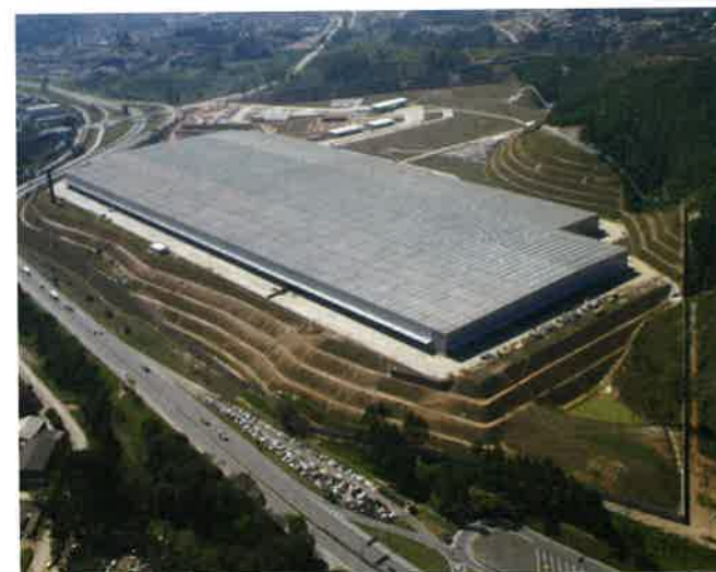
Figure 2.3.6-5 Industrial Building Provided with a Post-Tensioned Ground-Supported Slab (Brazil; Aereas; P375)
