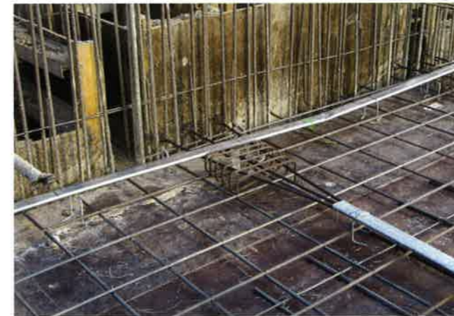
FIGURE 2.5.2A-9 Most Common Dead End Configuration (P174a)
