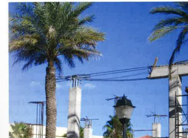
(b) Beam under construction (P665)
