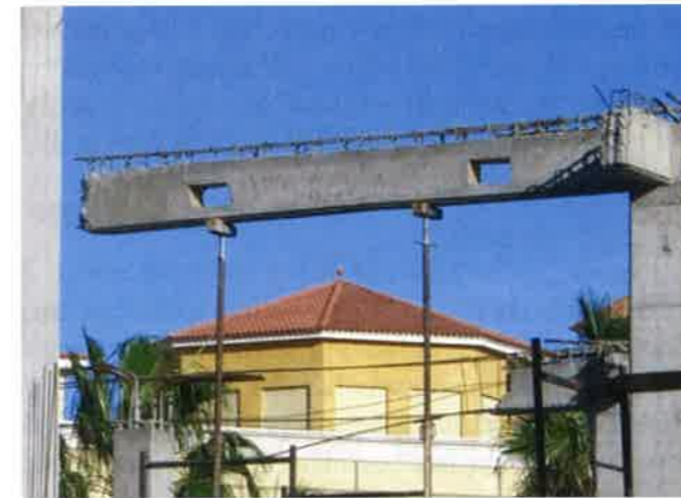
(a) Beam under construction (P664)
