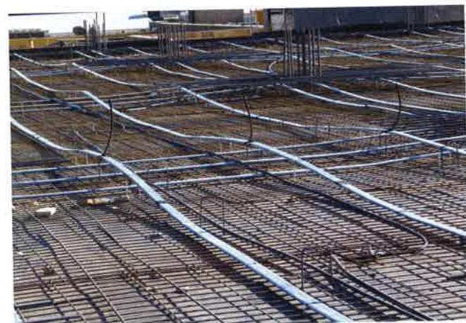
FIGURE 2.5.2-2 Grouped/Distributed Tendon Layout (P165a)
