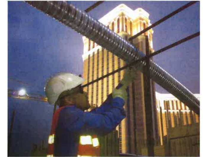
FIGURE 2.3.4-6 Technician Adjusting a Post-Tensioning Tendon for the Full 3.5 m (11' 6") Height (P365)
