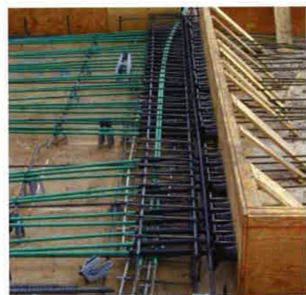
(c) Banded unbonded tendons in place with bursting bars (P594)
