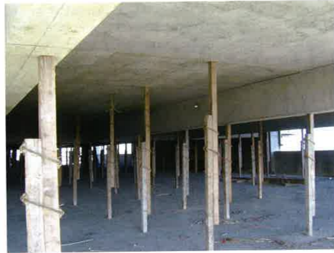
FIGURE 2.5.1L-2 Re-shoring of Beam and Slab Construction (P448)
