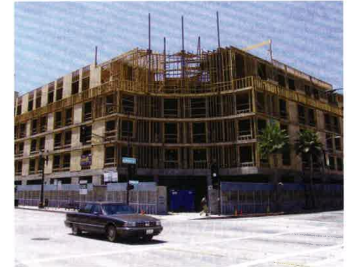
FIGURE 2.3.3-1 Low Rise Building with Post-Tensioned Podium Slab under Construction (California; P359)
