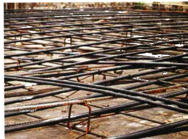
(b) Tendon Layout; Distributed-Distributed Arrangement (Thailand; P546)
