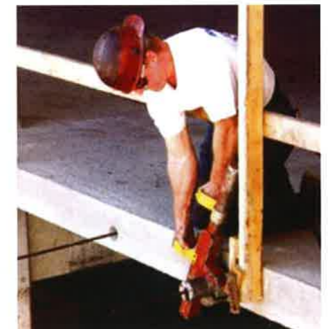
(b) Pocket shear in operation (P453)
