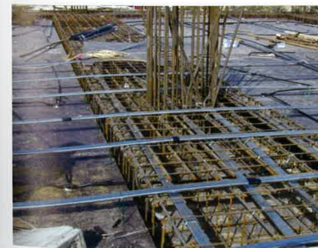
FIGURE 4.6.2-4 Construction View of a Slab Band Using Grouted Tendons (P285)
