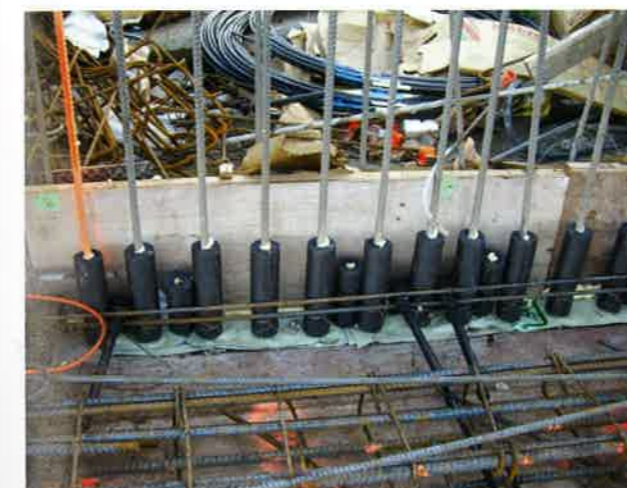
(b) Provision for release of a continuous wall (P312)
