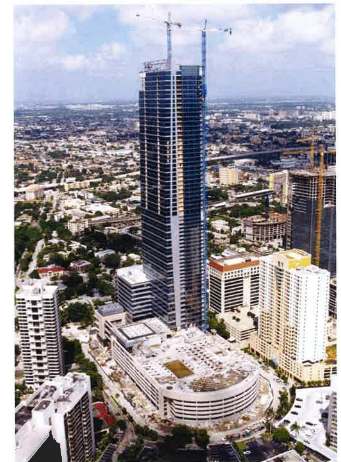
FIGURE 2.3.1B-1 Post-Tensioned Building Constructed to Resist Wind Forces (Four Seasons Hotel, Florida, P349)
