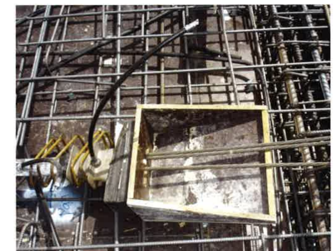
FIGURE 2.5.2C-2 Close up of a Stressing Pan at Top of Member (P180)
