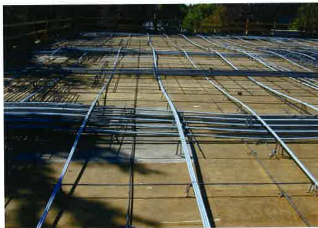
FIGURE 2.5.1-1 View of a Floor System Reinforced with Unbonded Tendons (P408)
