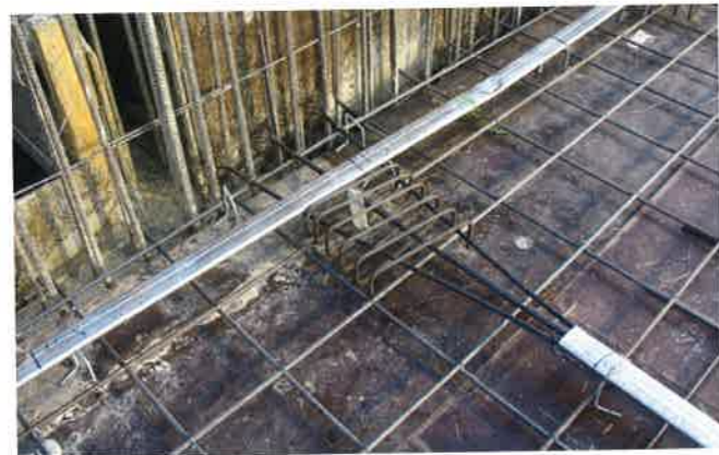
FIGURE 2.5.2C-4 Anti-Bursting Reinforcement behind Anchorage Device (P183)
