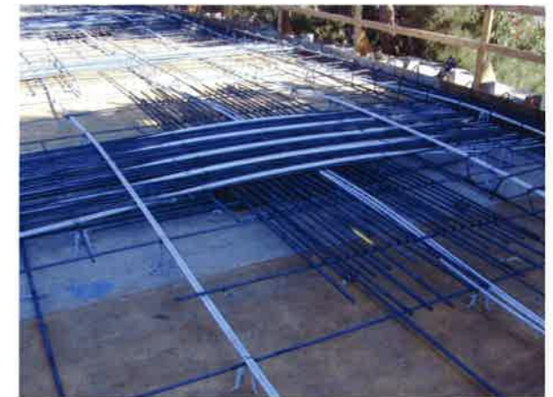
FIGURE 4.10.2A-6 View of Tendon Layout Showing the Position of Tendons Over Column (P564)
