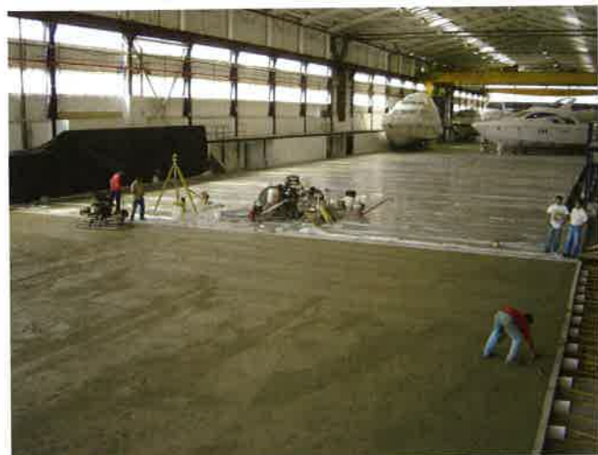
FIGURE 2.3.6-4 Industrial Floor Foundation Being Prepared with Friction-Reducing Moisture Barrier (P373)
