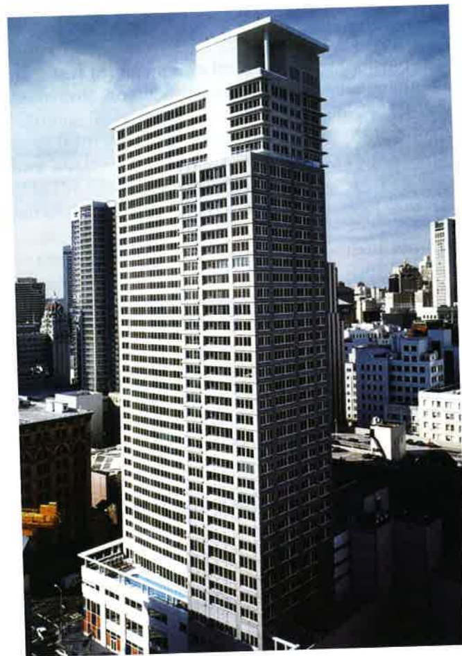
FIGURE 2.3.9-3 Paramount Building (San Francisco, California; P385)
