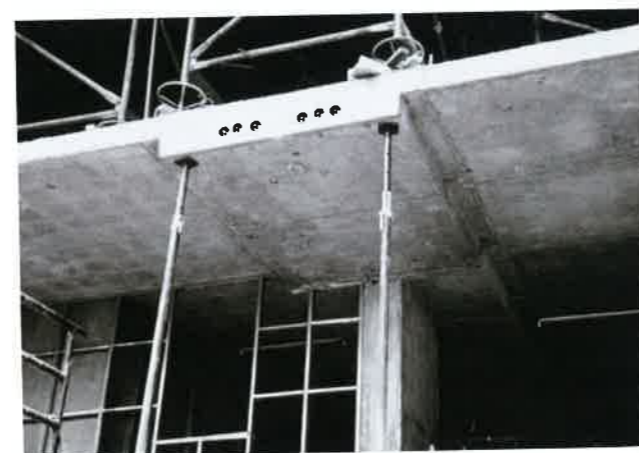
FIGURE 4.6.2-1 View of a Post-Tensioned Slab Band (P282)
