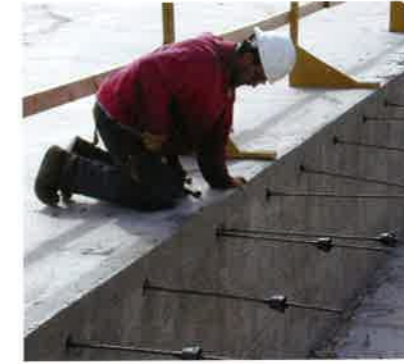
(b) Excess concrete is chiseled off (P435)
