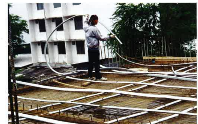
Figure 2.5.2A-6a Empty Flexible Ducts are Placed in Position (P172b)
