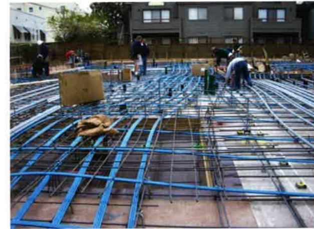
(a) Unbonded slab construction (P242)
