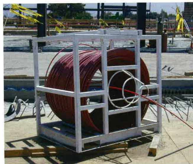
FIGURE 2.5.1A-2 Strand Delivered to Site in Coil (P403)
