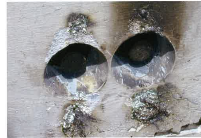
(a) View of capped stressing pocket (P260)
