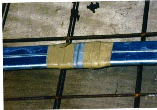
FIGURE 2.5.2C-5 Taped Duct Splice (P184)
