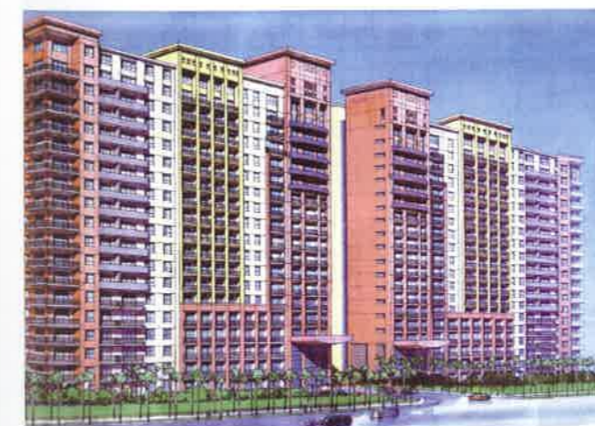
Figure 2.3.1A-4 Ocean Villa Apartments, Southern California (P348)
