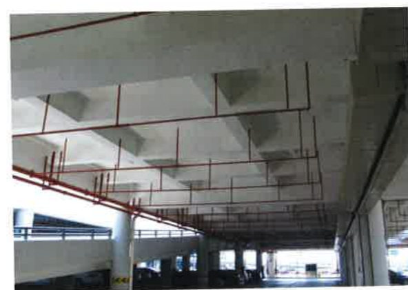
FIGURE 4.6.4A-4 Slab Panel Supported by a Square Grid of Beams (Hong Kong; P659)
