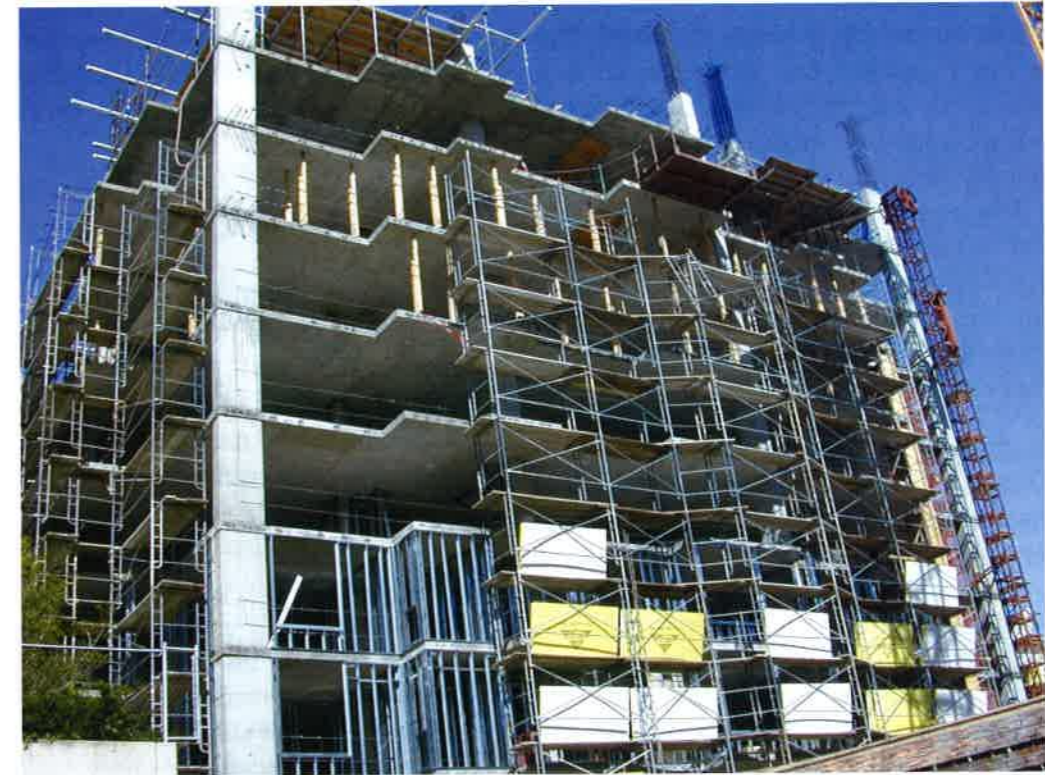
Post-Tensioned Building under Construction (US; P500)
