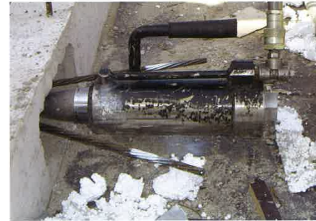
FIGURE 2.5.2G-1 Stressing Operation at Member Edge (P195)
