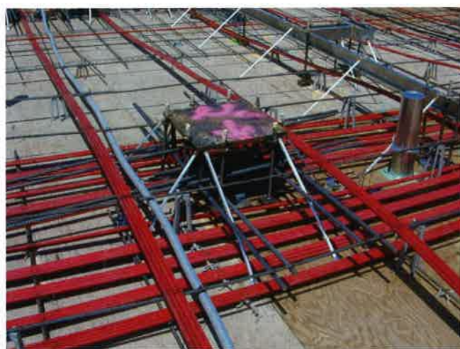
(a) Base plate of steel columns planted on PT slab (P136a)
