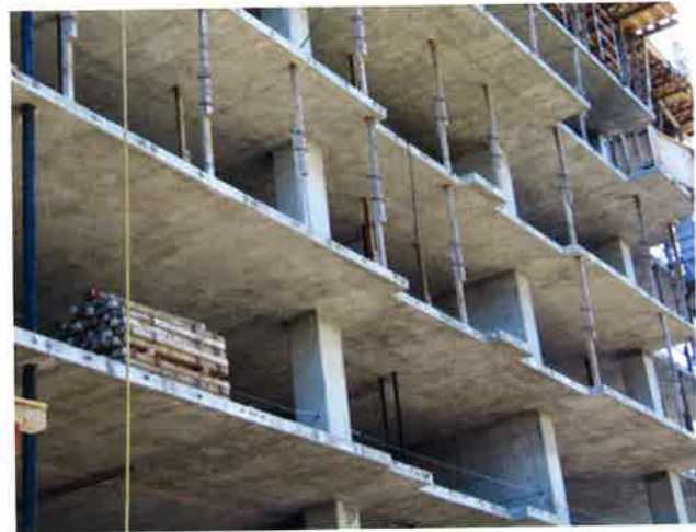
FIGURE 4.6.8-1 View of a Typical Post-Tensioned Flat Slab Construction in California (P314)
