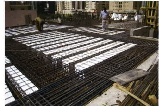
FIGURE 4.6.1B-4 Example of a Conventionally Reinforced Flat Slab Construction Using Foam Infills (Ryadh KSA; P280)
