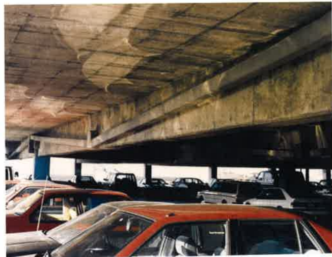
FIGURE 2.3.8A-4 External Tendon for a Continuous Beam (Pier 39 Parking Structure, San Francisco; P490)
