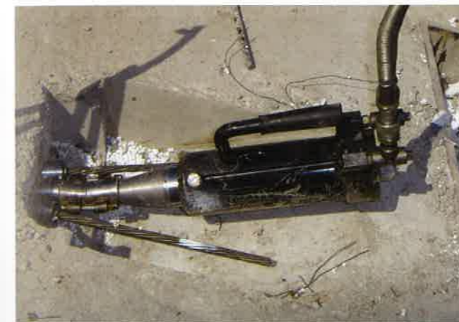
FIGURE 2.5.2G-2 Stressing Operation at Member top Surface (P196)
