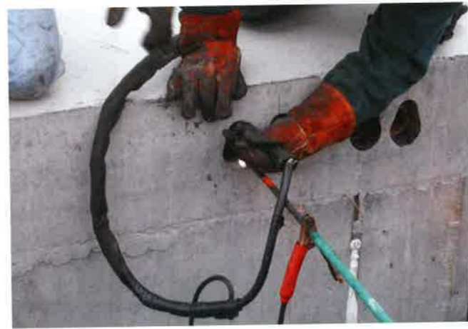
(b) Cutting strand tail using plasma cutter (P455)
