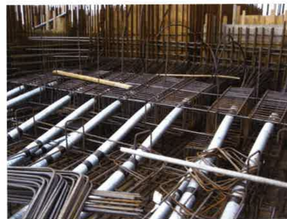
(b) Bursting steel arranged behind dead end of multi strand transfer plate (Macau; Freyssinet) (P596)
