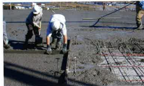
(b) Concrete is finished with a flat surface (P432)
