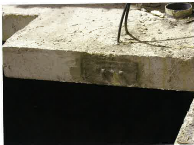
FIGURE 2.5.2K-1 Stressing Pockets are Sealed Off to Avoid Spilling at Grouting (P201)
