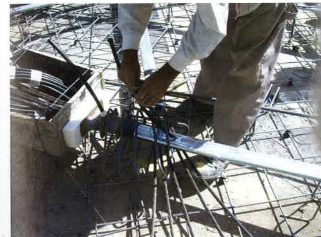
FIGURE 2.5.2C-9 Air Vent Tubes are Provided at Tendon Ends (KSA; P190)
