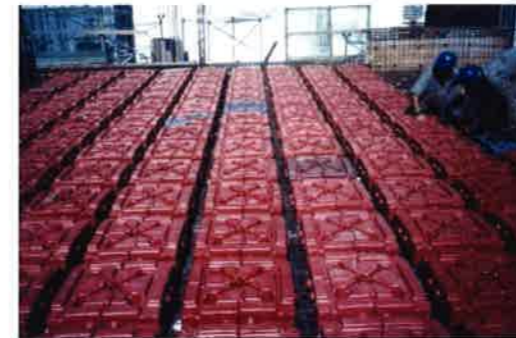
(a) Floor slab with plastic void generators (P279a)
