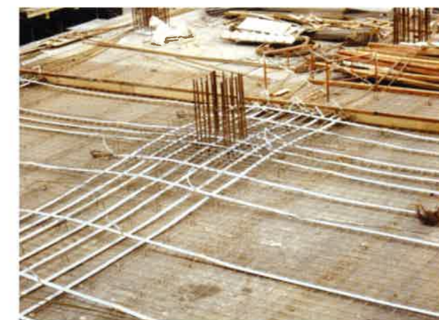
FIGURE 4.8.8A-4 Tendon Layout, using Banded-Distributed Arrangement (Grouted Tendons Singapore) (P545)
