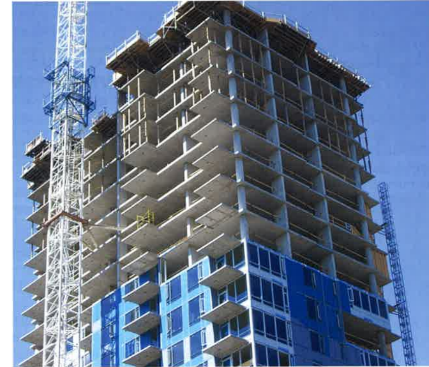
View of a Post-Tensioned Building (Seattle, USA, P133)
