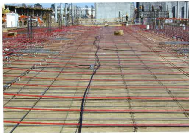
(b) Distributed tendons placed parallel (P424)
