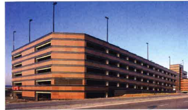
FIGURE 2.3.2-3 San Jose California International Airport Parking Structure (P357)
