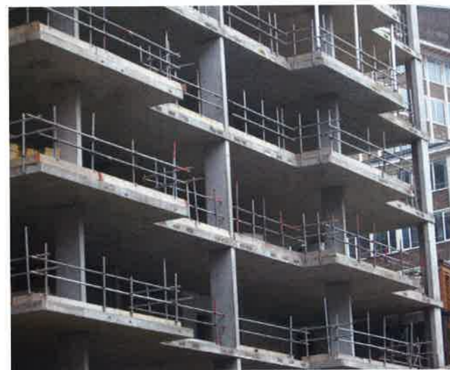
FIGURE 2.3.1C-2 Post-Tensioned Building (Knightsbridge, London; P354)
