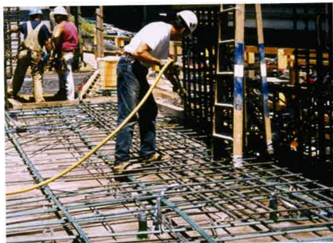
FIGURE 2.5.1F-2 Air Pressure is used to Blow out Loose Debris (P430)
