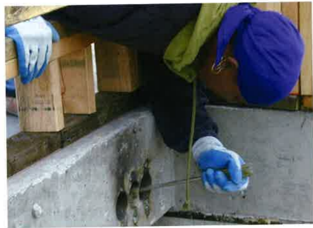
(a) Excess material is removed from recess block (P456)
