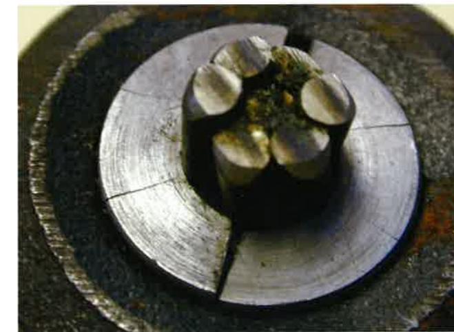
FIGURE 2.5.1J-3 Cracking of Wedges at Stressing (P446)
