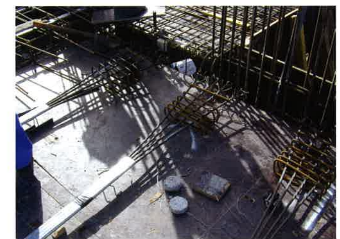
(b) Dead end anchorage of a flat duct (P146b)
