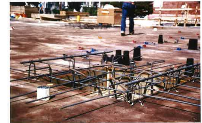
(b) Heavy bars on two sides of a support (P407)
