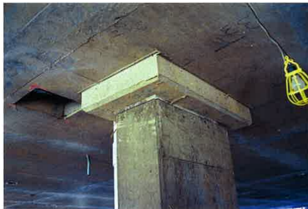
FIGURE 4.11.6.6-1 Opening Near a Column Support (P637)
