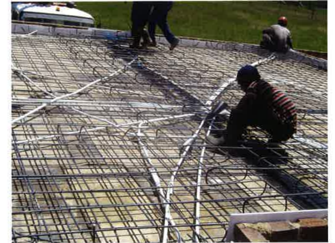
(a) View of a conventionally reinforced slab (P138)
