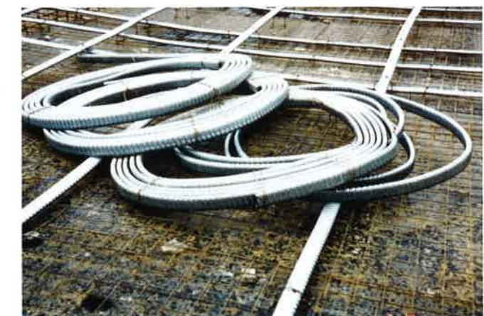
2.5.2A-5 Bundle of corrugated Ducts Ready for Installation (P172a)
