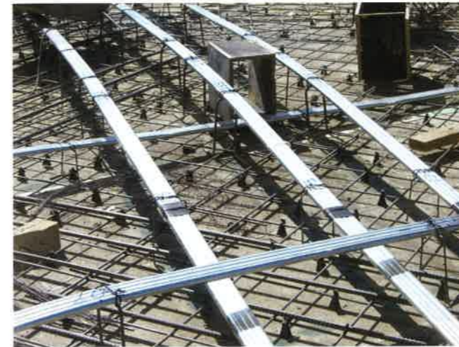
FIGURE 2.5.2C-8 Individual Chairs Create the Design Profile (P189)
