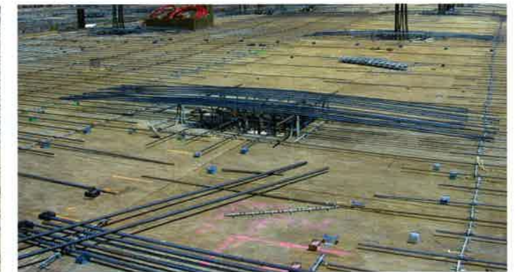
(b) Bottom bars at exterior spans (P415)
