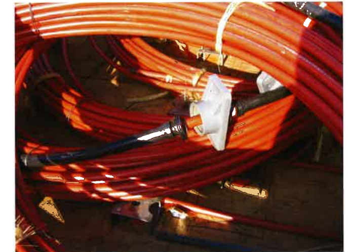
FIGURE 2.5.1A-4 Anchors for Intermediate Stressing are installed in the Shop (P405)
