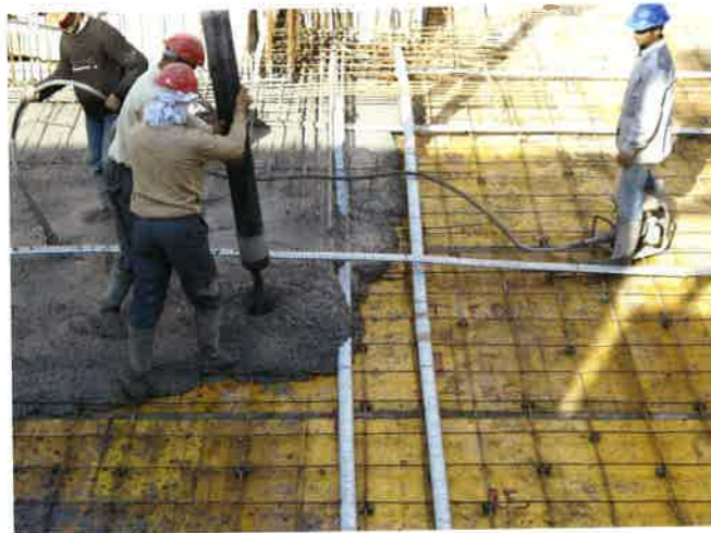
FIGURE 2.5.2E-1 Placing of Concrete (P192)
