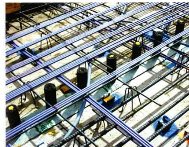
(a) Provision for release of a discontinued supporting wall (P311)
