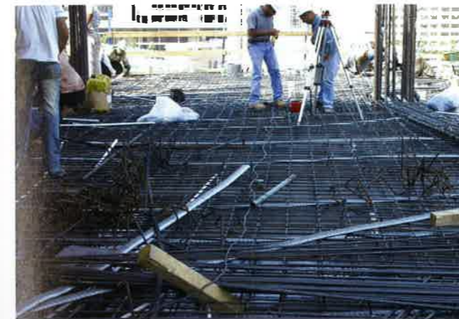
FIGURE 2.5.2C-1 Tendon are Threaded through Installed Non-prestressed Reinforcement (Dar Al-Handasah Beirut; P178)
