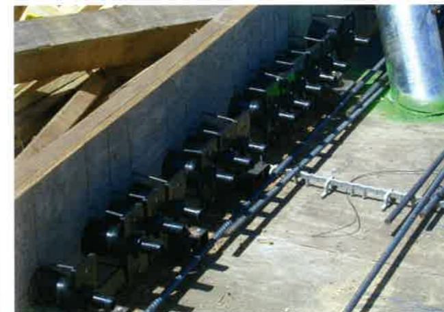
FIGURE 2.5.1C-1 Stressing Ends at the Slab Edges (P416)
