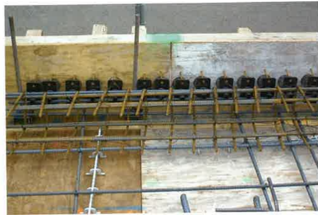
(a) Live ends are secured to the bulkhead and provided with anti-bursting reinforcement (P419)
