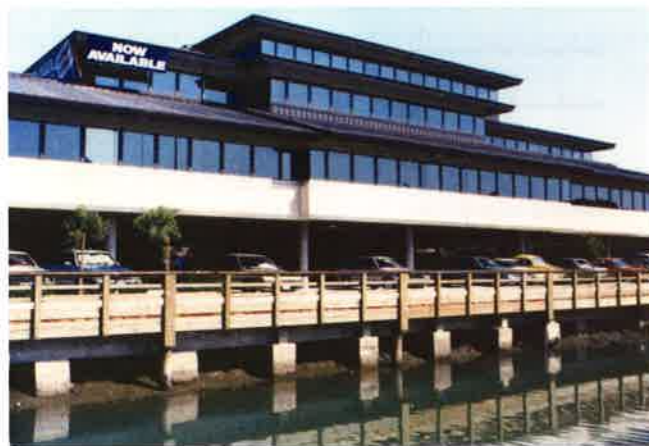
(a) Office building constructed with steel framing on a post-tensioned slab (P137a)
