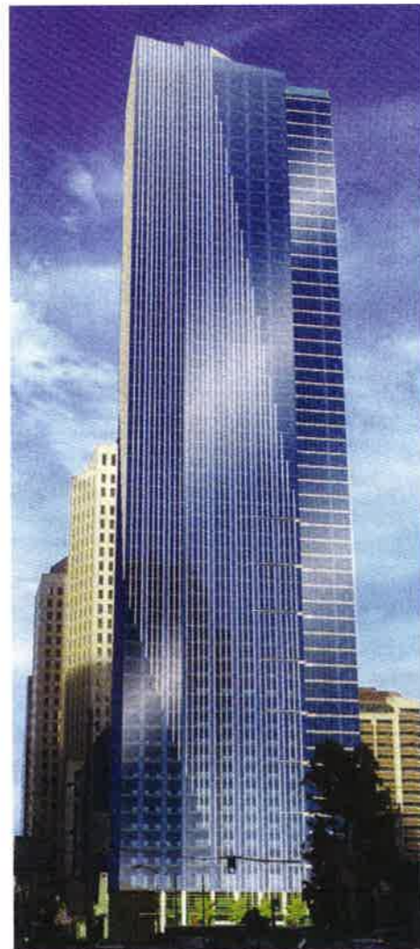
FIGURE 2.3.1A-1 Post-Tensioned Building at 301 Mission Street, San Francisco, California (P342)
