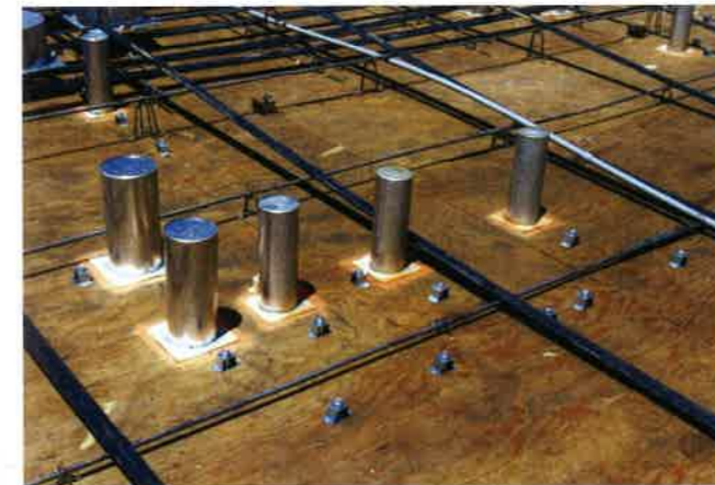
FIGURE 2.5.1D-1 Inserts for Plumbing and Other Utilities (P525)
