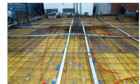
FIGURE 4.8.8C-1 Tendons Spaced More than 5 Times Slab Thickness (Morocco; P550)
