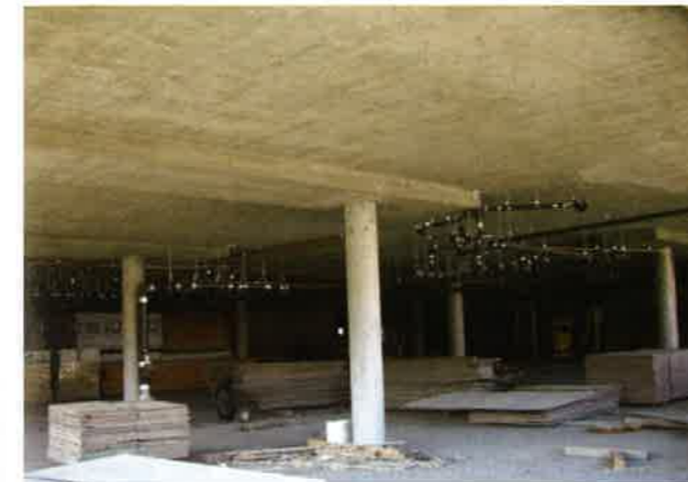
FIGURE 4.6.2-2 View of a Slab Band Extending Over the Long Spans (P283)
