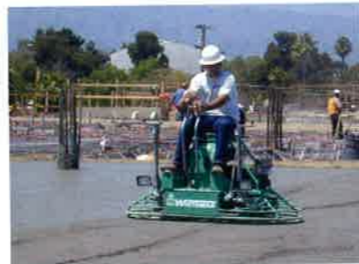
(c) Rotary trowler is used for a smooth surface (P433)
