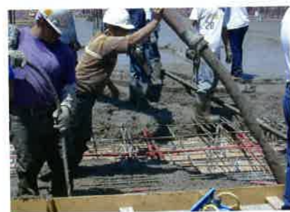
(a) Concrete is pumped and consolidated (P431)
