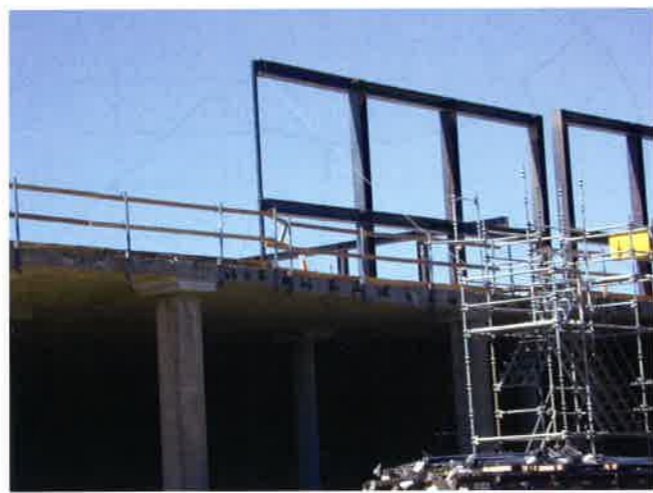
(b) Steel frames planted on post-tensioned slab (P136b)
