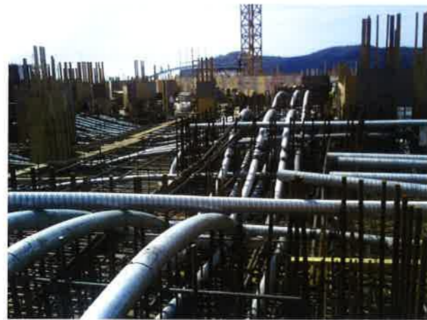
FIGURE 4.11.6.4-5 Reinforcement Installation of a Transfer Plate (Freysinet HK; P705)
