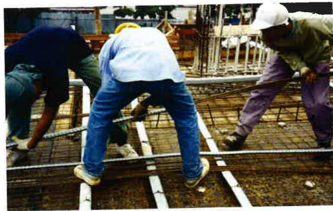
FIGURE 2.5.2A-6b Strands are Pushed into Positioned Ducts (P173)
