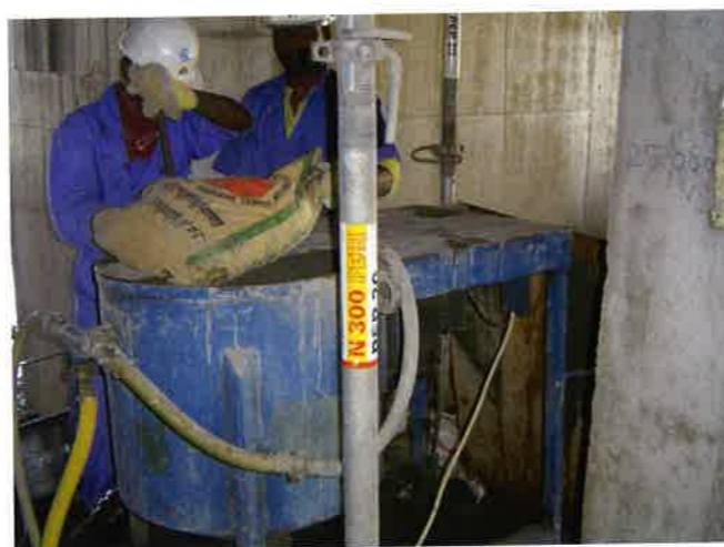
FIGURE 2.5.2K-2 Grout Mixer Using Pre-mixed Bags (P202)
