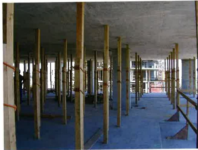
FIGURE 2.5.1L-1 Re-shoring of Flat Slab Construction (P447)
