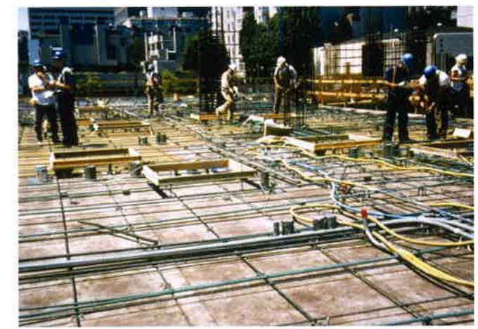
FIGURE 2.5.1E-1 Inspection by Trades Involved Prior to Placing of Concrete (P428)
