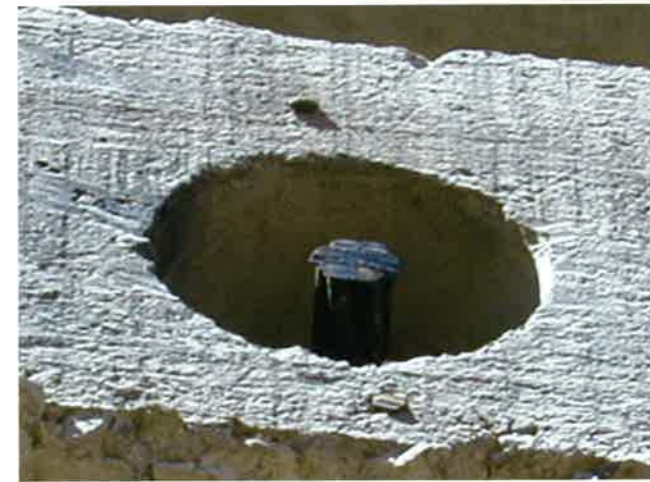
FIGURE 2.5.1M-2 Cutting of Strand Tail, Using Abrasive Saw (P451)
