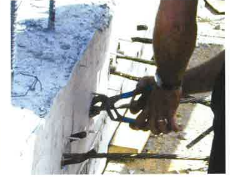
(c) Pocket formers are removed (P436)
