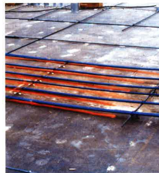
(a) Spray paint on form at low point region of tendon (P205a)
