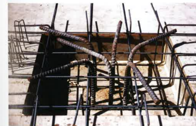
(a) Column drop reinforcement (P406)
