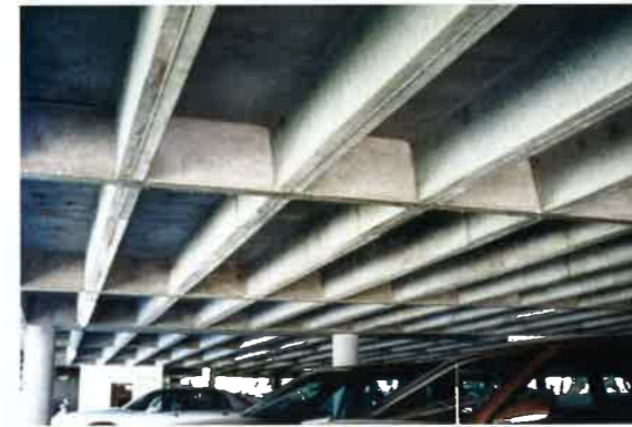
FIGURE 4.6.5-1 View of a Joist Slab Construction (P295)
