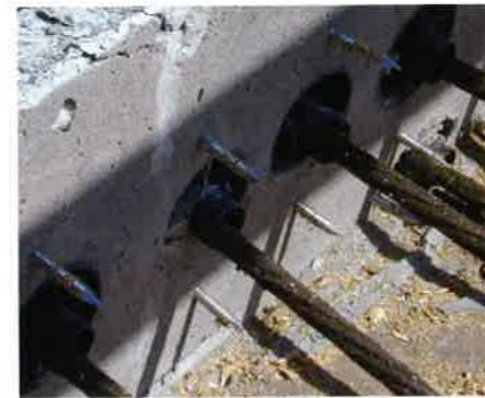
(a) Form is removed from slab edge (P434)
