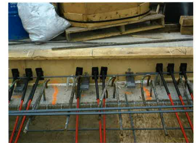
FIGURE 2.5.1C-3 Dead Ends are Positioned 2" (50 mm) from the Bulkhead (P418)
