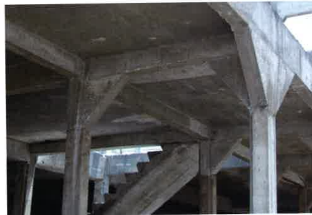
(b) Completed framing and floor slab (P317)
