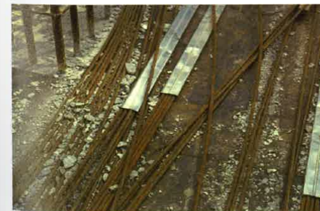
FIGURE 2.5.2A-3 Strands are pushed through the Ducts, Preparing the Tendon for Installation (P170)
