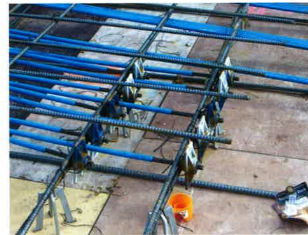
FIGURE 4.4.1.3-1 Example of Application of a post-tensioning System in Use in a "Non-Corrosive" Environment (P501)
