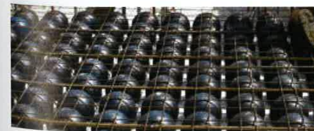
FIGURE 4.6.1B-3 Voided Slab Construction (P278)
