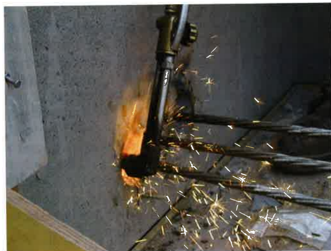
(a) Flame to cut strand tail (P449)
