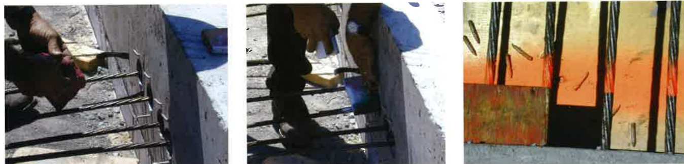
(c) View of datum marks on tendon tails (P442)
