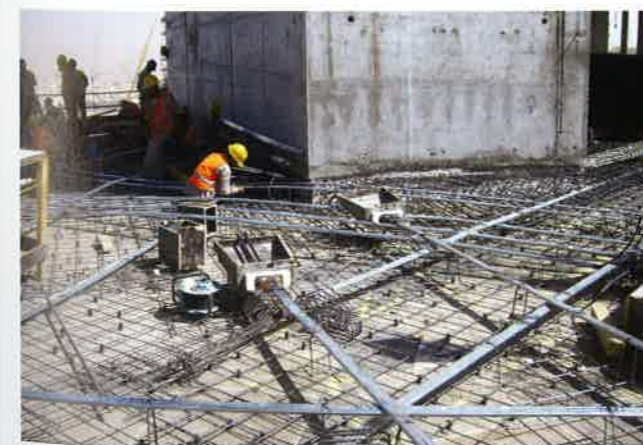
FIGURE 2.4-6 Grouted System Construction in Progress (KSA; P473)
