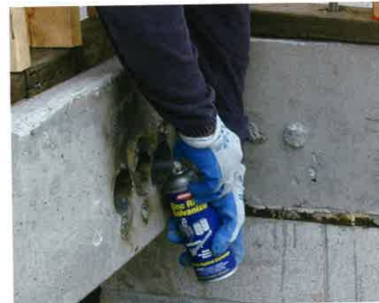
(b) A corrosion inhibiting spray, such as Zinc-based galvanizer is used for added protection (P457)
