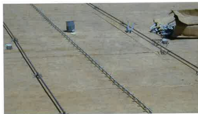
FIGURE 2.5.1B-4 Support System for Distributed Tendons (P413)
