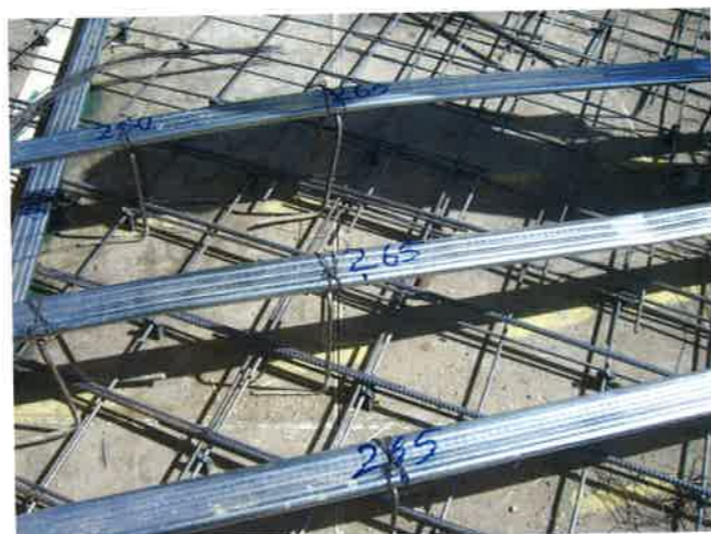
FIGURE 2.5.2C-7 Required Chair Heights are Marked along the Length of Each Tendon (P186)
