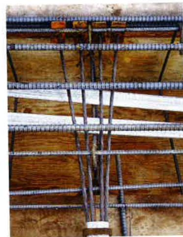
(b) Single anchorage castings used as anchorage device (P513)
