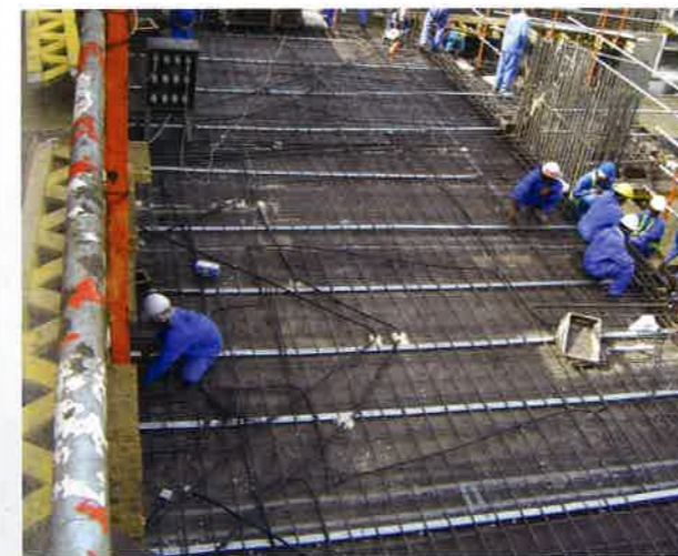
(a) One-Way Floor System (JBR) Dubai, grouted (P508)
