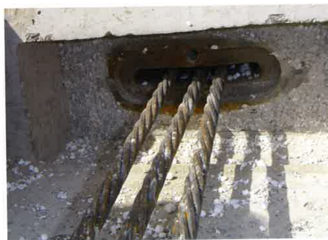
FIGURE 2.5.2F-1 Anchorage Device Ready to be Stressed (P194)
