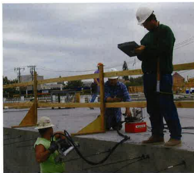
(a) Stressing equipment and crew (P443)
