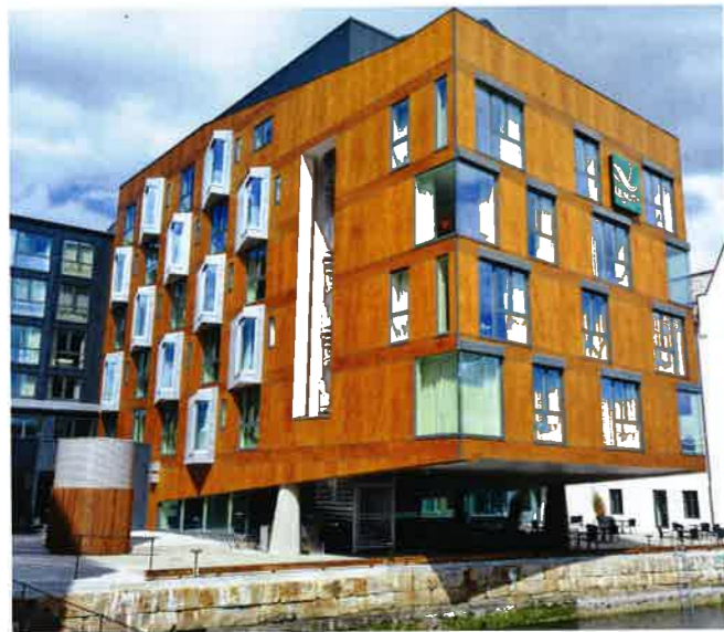
FIGURE 2.3.1C-1 Post-Tensioned Building Aslund (Norway) Cantilevering over Promenade (P353)
