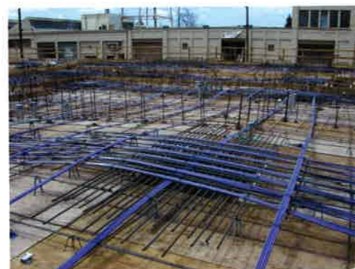
FIGURE 4.8.8D-3 Banded Tendon Pressed Against Top Reinforcement Grid (P339)
