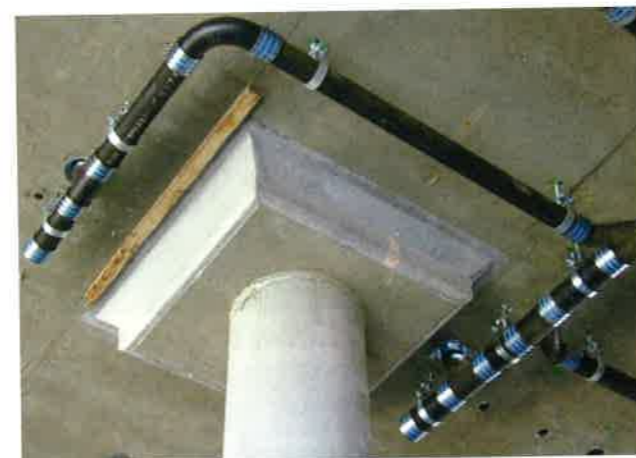
(a) View of a square column drop used for punching shear (P286)
