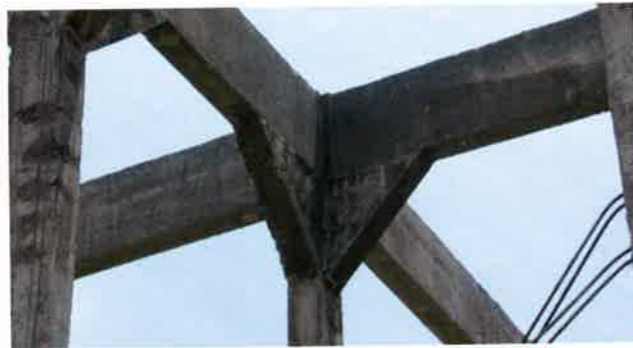
(a) Framing to support floor slab (P316)
