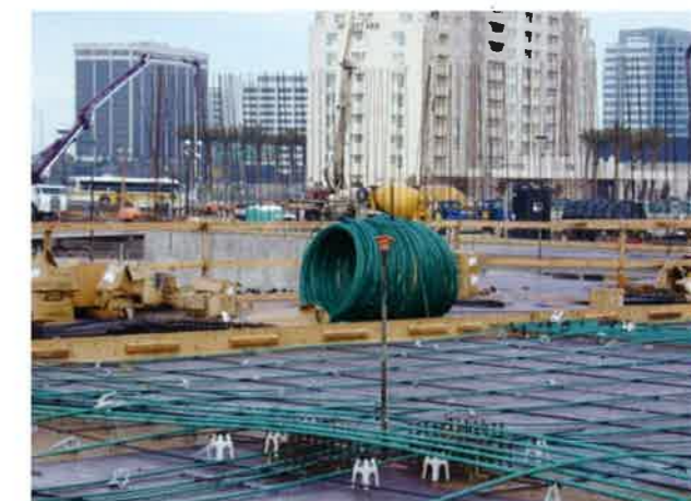
FIGURE 4.8.8A-3 View of Banded-Distributed Layout (Unbonded tendons; UK; P548)
