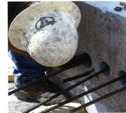
(b) Wedges are inserted in anchorage casting (P438)
