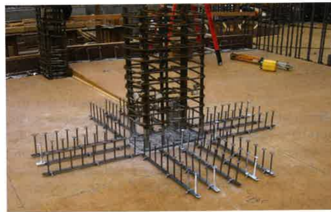
(b) Installation of shear reinforcement (P412)
