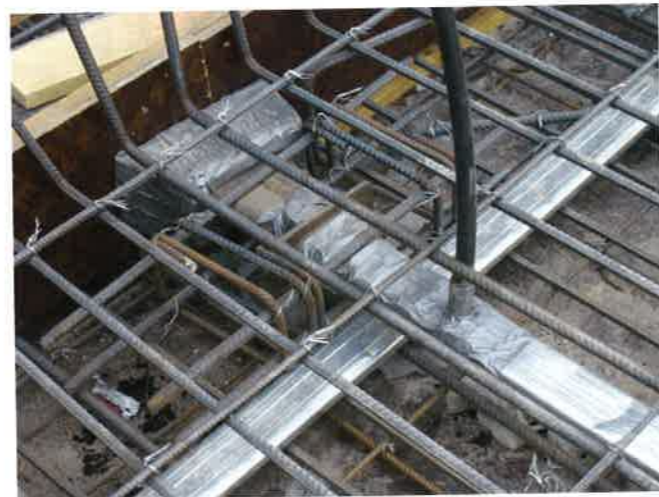
FIGURE 2.5.2C-6 Pocket Former for Stressing using Tape Over Styrofoam (MEPS; P185c)
