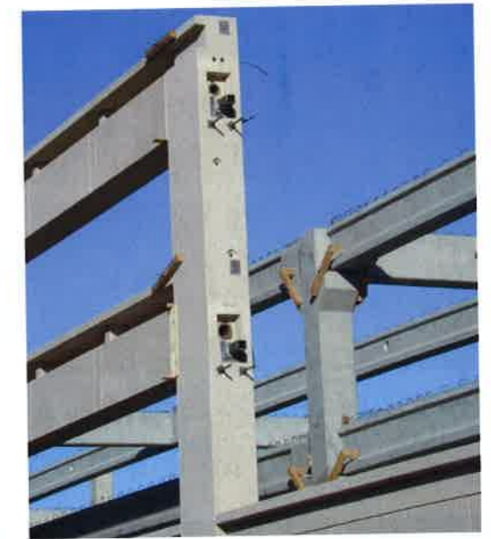
(b) Close up of frame showing tendon duct (P387b)
