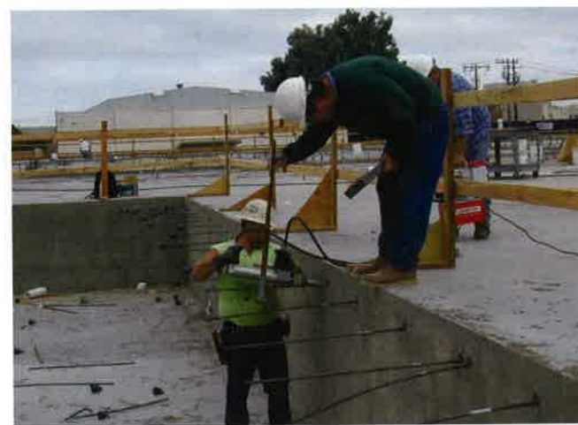
(b) Elongation measurement by inspector (P444)
