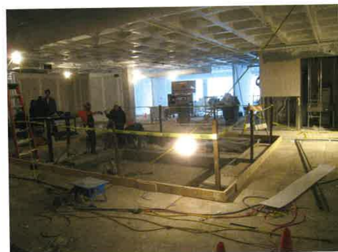
(a) View of floor system and stairwell opening (P478)
