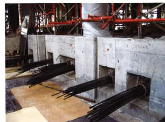
(b) Tendons at slab edge were subject to stage construction (P369b)
