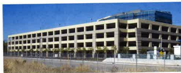
(b) View of a parking structure (P301)
