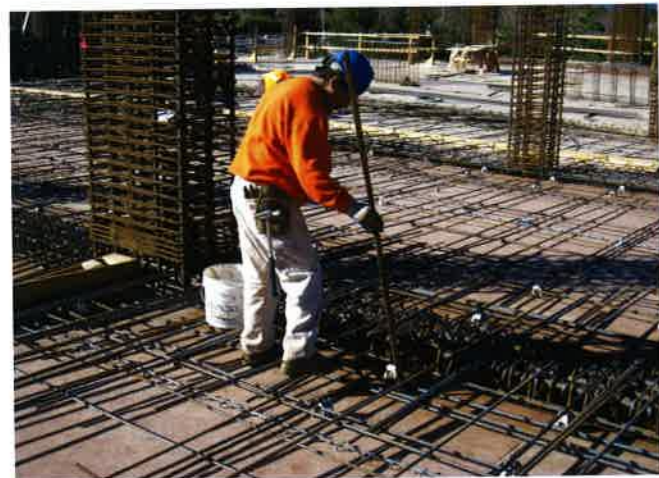
FIGURE 2.5.1F-1 Form is Swept with a Strong Magnet to Collect Loose Nails and Wire (P429)
