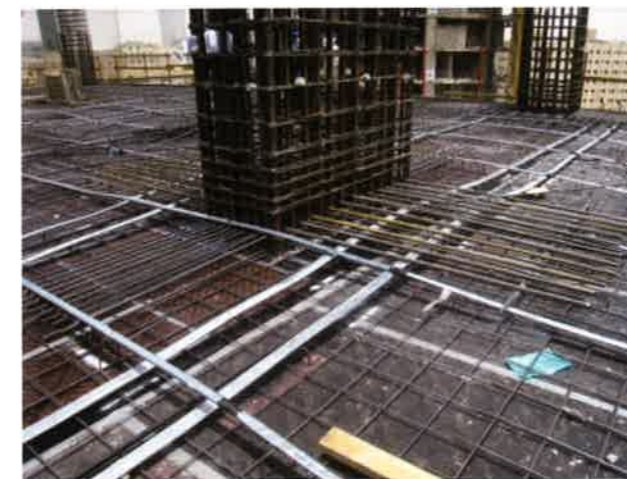
(b) Grouted slab construction (P243)
