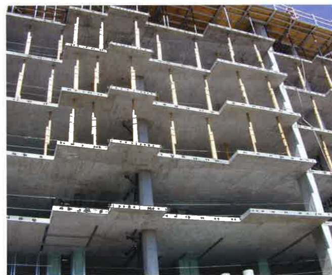
FIGURE 2.2E-1 Beamless Flat Slab Construction Using Post-Tensioning (P134)
