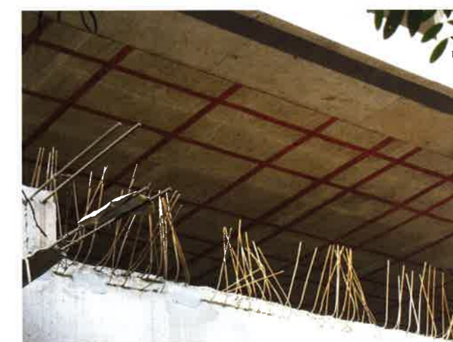
FIGURE 2.5.3A-2 Soffit of Slab is Painted to Show the Location of Tendons (Mumbai; P206b)
