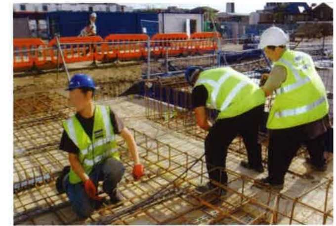
FIGURE 2.5.2A-4 Strand is Pushed into an Installed Duct (P171)
