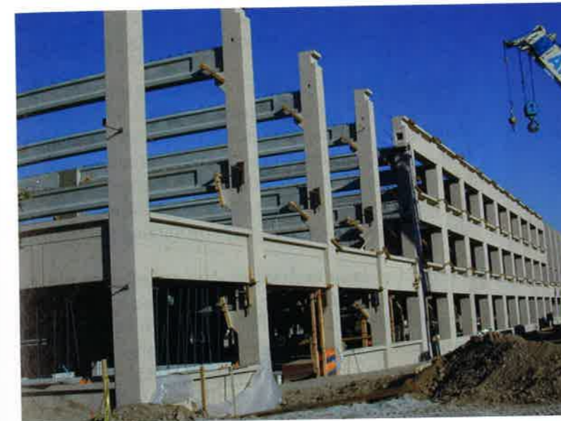
(a) Partially assembled frame (P387a)
