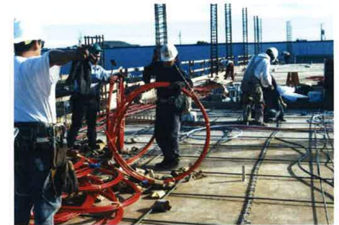
FIGURE 2.5.1C-2 Tendons are Unrolled and Placed (P417)
