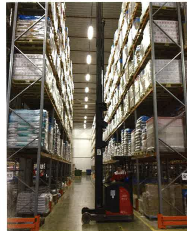
FIGURE 2.3.6-1 Industrial Floor Slab with Storage Stacks Served by Forklift Trucks (Courtesy ADAPT; Moscow; P717)
