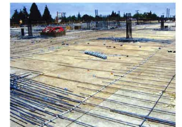
FIGURE 4.10.2A-8 View of Bottom Bars, Staggered by 12" (300 mm) (P241)
