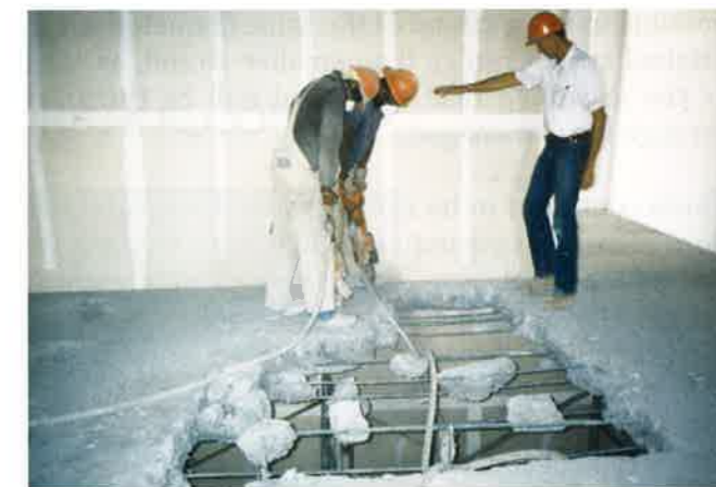
FIGURE 2.7.2-3 Removal of Concrete around Tendons (P480)
