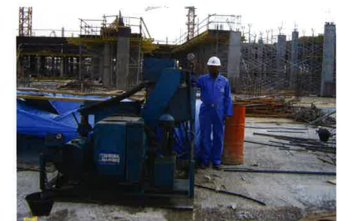
FIGURE 2.4.4-1 View of Grouting Equipment (P162)
