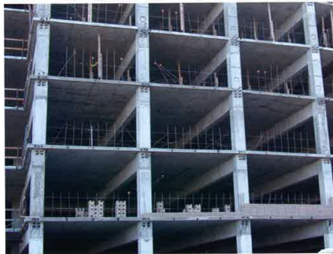
FIGURE 2.3.2-1 View of Rostam Parking Structure (P355)
