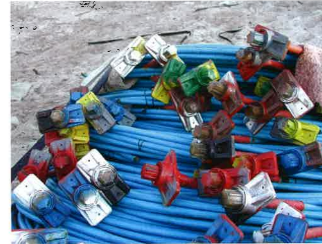
FIGURE 2.5.1A-3 Shop Fabricated Tendons are Color-Coded and Tagged (P404)
