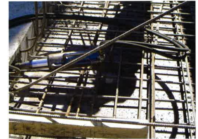
(b) Strand threads through jack (P159b)
