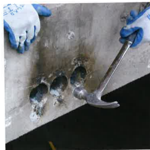
(d) The cap is hammered (screwed) in position (P459)
