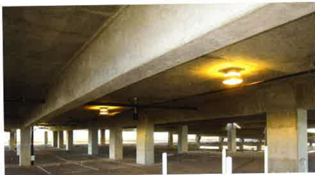
(a) Interior view of a beam and one-way slab construction (P300)
