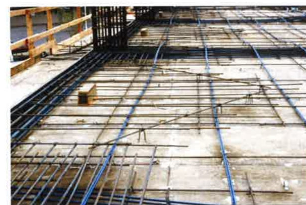
(b) Reinforcement between grouped tendons (P327)
